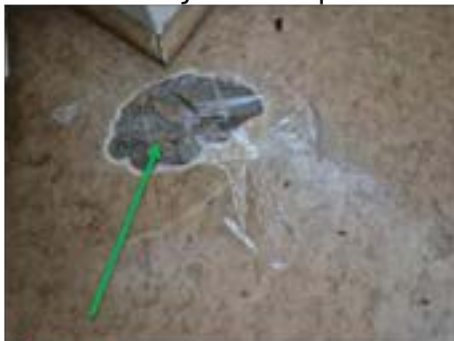
✓ 11003:2 Svartlim + underlagspapp under linoleum. Ej asbest.
