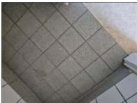
✓ 10011:2+10036:2+12030:2. Fog vitt kakel. Ej asbest.
