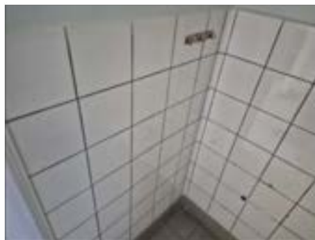
✓ 10011:1+10036:1+12030:1. Fog vitt kakel. Ej asbest.
