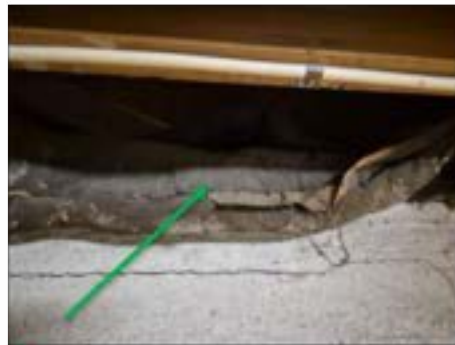
✓ Vind:3. Runt isolering. Papp. Ej asbest. Ej PAH.
