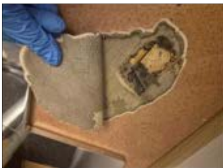
✓ 12036:1 Svartlim under dold linoleum. Ej asbest.
