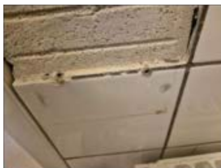
✓ 10045:1. Fog vitt kakel. Ej asbest. Ej asbest.
