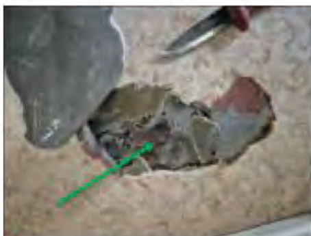
✓ 12005:1. Mörkbrunt lim under dold linoleum. Ej asbest.
