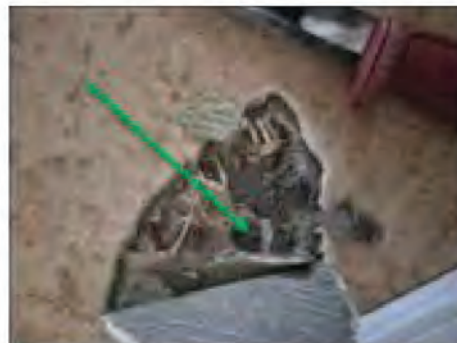
✓ 10019:1 + 10022:1. Under dold linoleum Underlagspapp+svartlim. Ej asbest.
