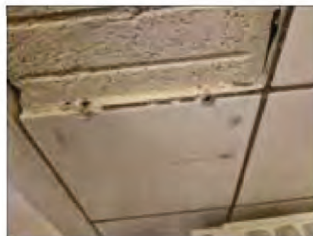
✓ 10045:1. Fog vitt kakel. Ej asbest. Ej asbest.
