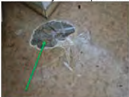
✓ 11003:2 Svartlim + underlagspapp under linoleum. Ej asbest.
