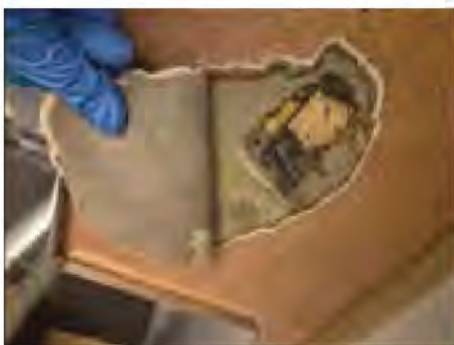
✓ 12036:1 Svartlim under dold linoleum. Ej asbest.
