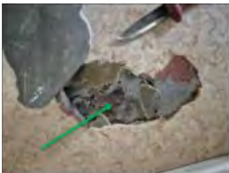
✓ 12005:1. Mörkbrunt lim under dold linoleum. Ej asbest.
