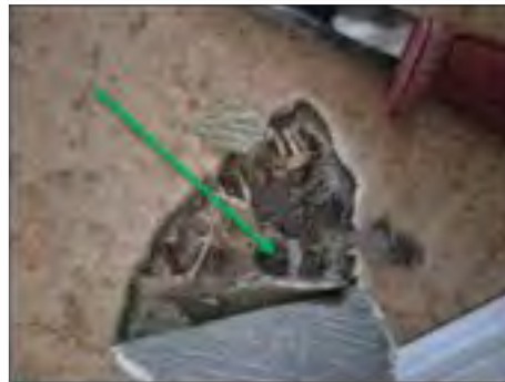
✓ 10019:1 + 10022:1. Under dold linoleum Underlagspapp+svartlim. Ej asbest.
