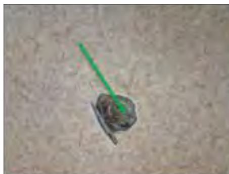
✓ 10042:1+12018:1. Mörkbrunt lim under dold linoleum. Ej asbest.
