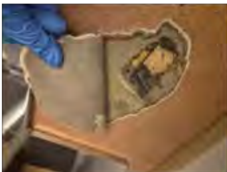
✓ 12036:1 Svartlim under dold linoleum. Ej asbest.
